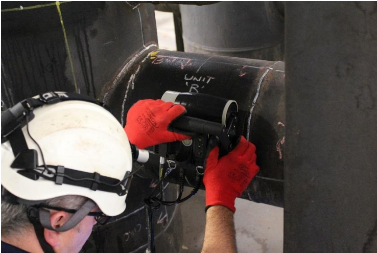
Figure 1 – WP128 inspecting the full circumference of a straight pipe section.
