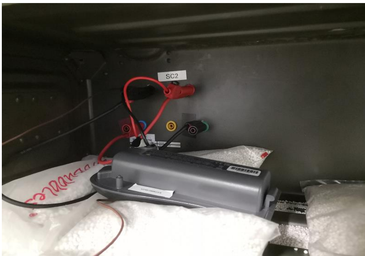
Picture 12: Sample connected to short circuit contactor
